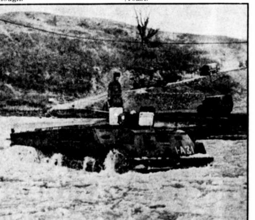
**CRACKER TRACK**—A U. S. Marine Corps amphibious "Tractor" breaks an ice jam in a Korean river to keep vital supplies rolling over a pontoon bridge to Canadian front-line positions. Smashing ice, which would break up supply-route bridges, is one of the many tasks performed by this versatile new fighting vehicle.
