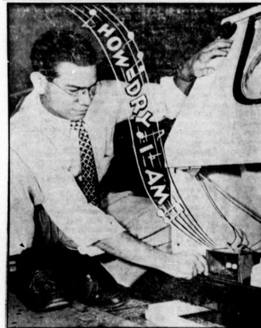
**HOT MUSIC BOX**—This electrically heated clothes dryer gives with a wail when wet wash is dry, thanks to inventiveness of William A. Wasmann of Mansfield, Ohio. The 30-year-old laundry-equipment creator rigged up the device that plays "How Dry I Am" at the end of each drying cycle. Wasmann earned his mechanical-engineering master's degree with a thesis on harmonics of vibrating strings, was assigned development of the musical attachment at Westinghouse's Electrical Appliance Division.
